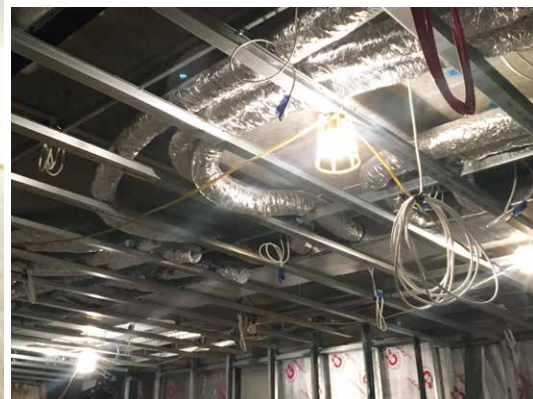
Above: Invisible.AC 25mm horizontal wall slot Below: Invisible.AC in-progress installation, requiring only 150mm ceiling void
