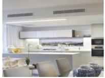
Ducted systems are usually a more expensive choice but are aesthetically pleasing. They can be used to cool multiple rooms, but you cannot have room control unless there is more than one system. The unit can be concealed in a false or suspended ceiling so that only a grille is visible.
